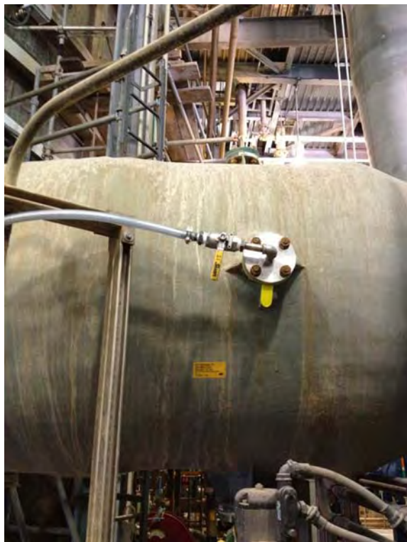
Recirculation Line Injection
